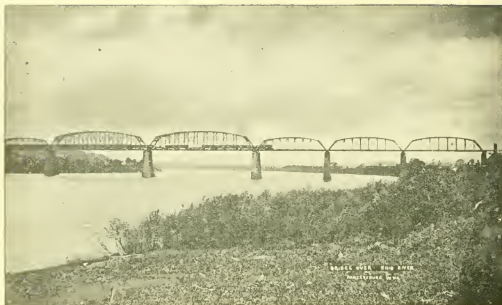
Baltimore & Ohio Bridge Over the Ohio River at Parkersburg.
